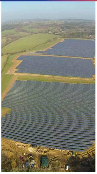
Solar farm constructed in Dorset, UK totalling near 7MW and 26,923 solar panels
